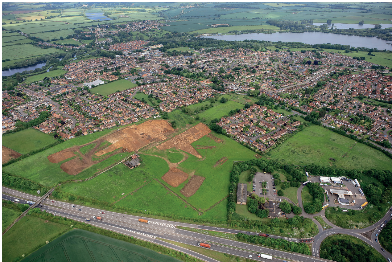
Plate 1.1: Aerial view of the development area with A14 in the foreground and Thrapston in the background, looking north-west
